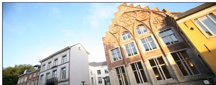
Faculty of Economics and Business Campus Leuven - Restored historical facade
